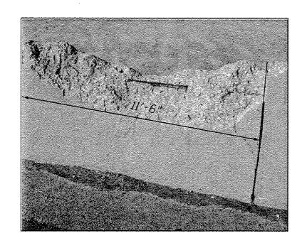
HALF DEPTH REPAIR REPLACE II½' OF BARRIER WALL FOR MORE DETAILS. SEE SHEET #6
