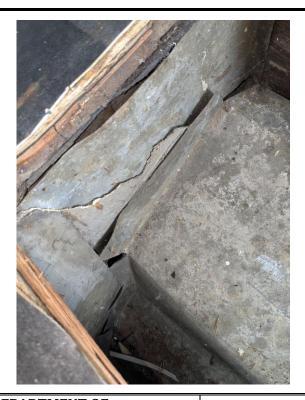
Material Description: Duct Wrap - Tested Positive for Asbestos
