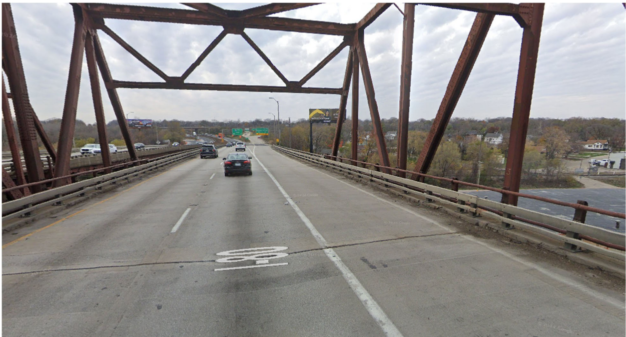
Exhibit 2c – Existing Site Conditions for Wall B24, looking West along I-80
