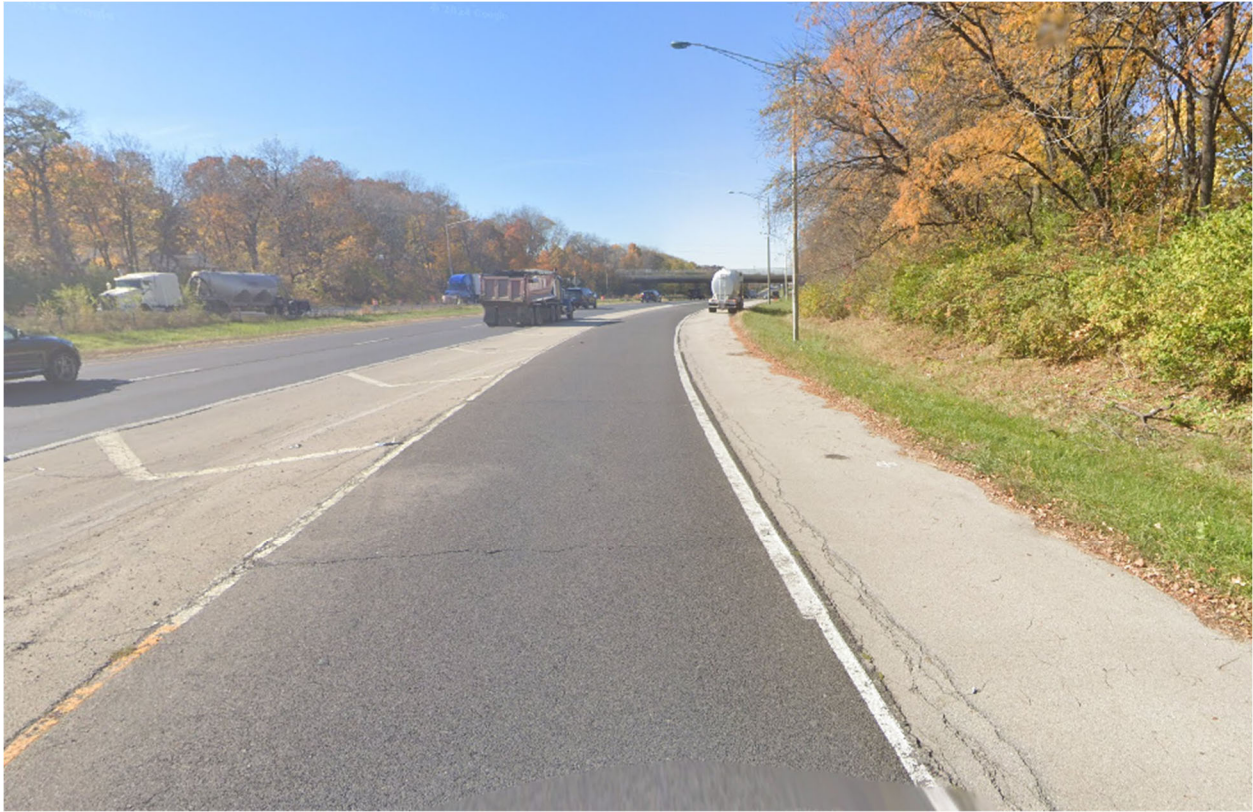
Exhibit 2b – Existing Site Conditions for Wall B23, looking West along I-80
