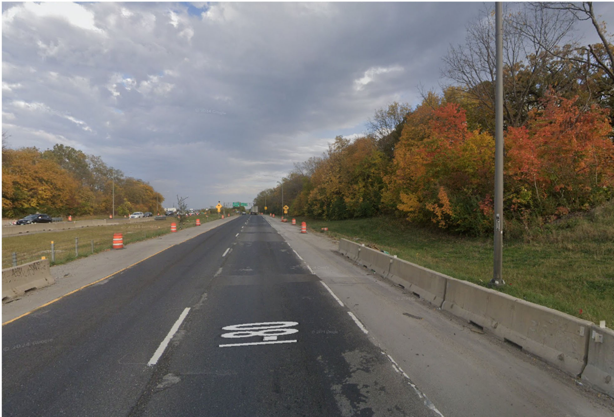
Exhibit 2a – Existing Site Conditions for Wall B22, looking East along I-80
