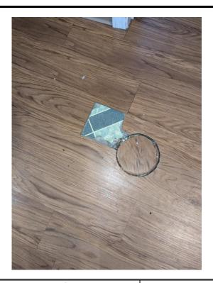
Material Description: Suspect ACM 12"x12" Blue with Light Blue Floor Tile & Mastic
