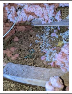
**Material Description:**Suspect ACM Vermiculite
