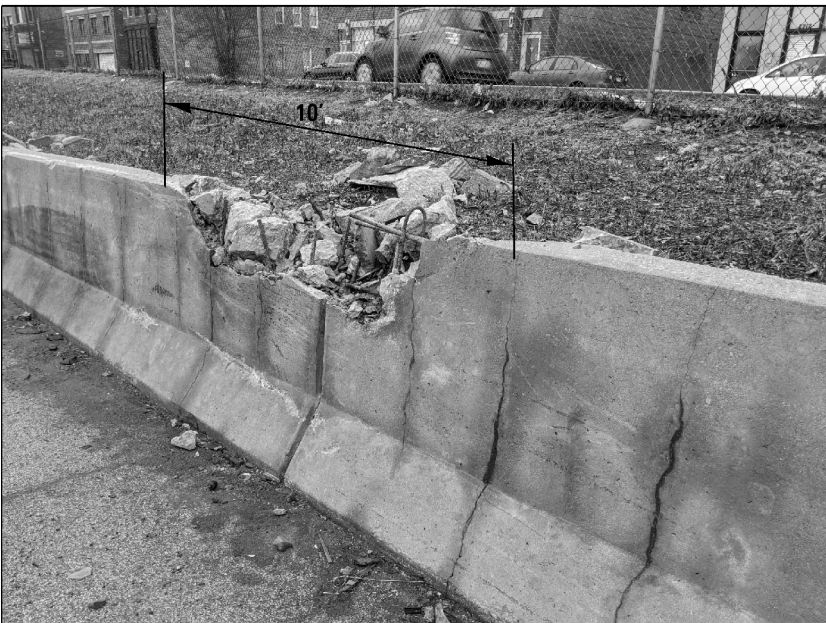
LOCATION 10. HALF DEPTH BARRIER WALL REPAIR REPLACE APPROXIMATELY 16 FT (2 SECTIONS) OF PARAPET LOCATED AT I-94 (DAN RYAN) SB LOCALS RIGHT SIDE JUST PAST 31st ST EXIT
