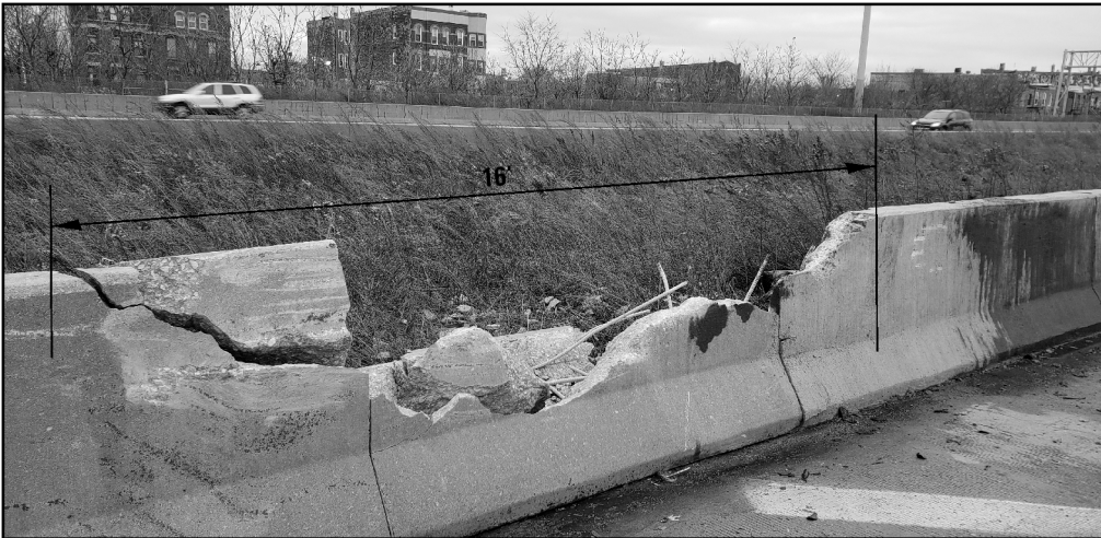
LOCATION 15. HALF DEPTH BARRIER WALL REPAIR REPLACE 16 FT OF PARAPET LOCATED AT I-55 SB AT APPROXIMATELY LOOMIS ST LEFT SIDE
