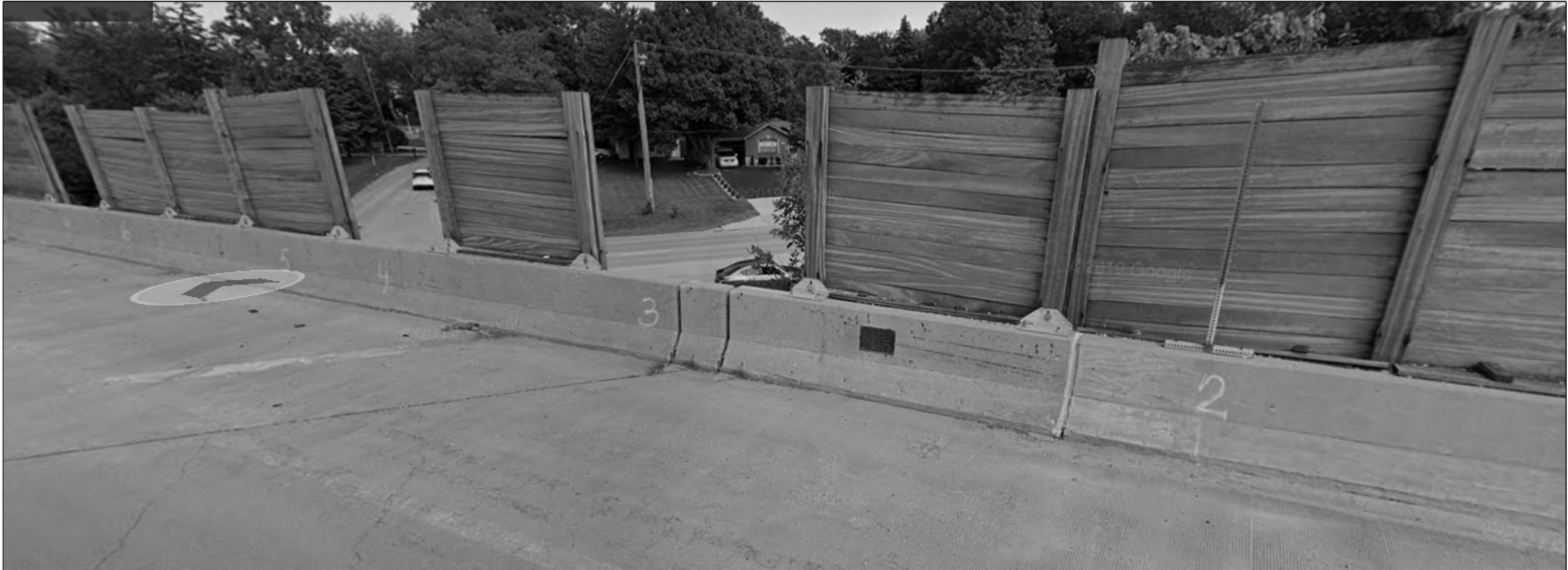
WOODEN NOISE WALL ON TOP OF CONCRETE BARRIER SEE LOCATION 21 SHEET 2 OF 2 FOR INFORMATION.
