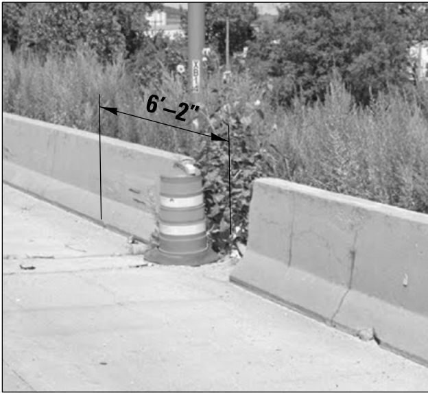
LOCATION 12B. FULL DEPTH PARAPET REPAIR REPLACE APPROXIMATELY 6'-2" OF PARAPET LOCATED AT I-94 (BISHOP FORD FWY) NB APPROXIMATELY 0.5 MILE OF DOLTON AVE RIGHT SIDE
