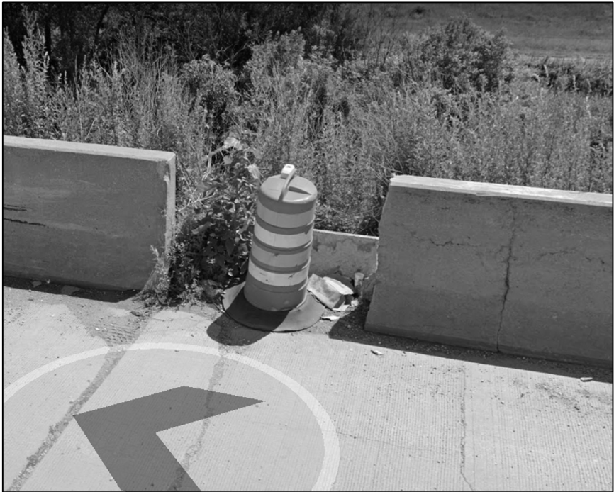
LOCATION 4B FULLL DEPTH BARRIER WALL REPLACE APPROXIMATELY 6 FT SECTION LOCATED AT EAST SIDE-100 FT NORTH OF TRUSS APPROACH SPANS ON ROADWAY
