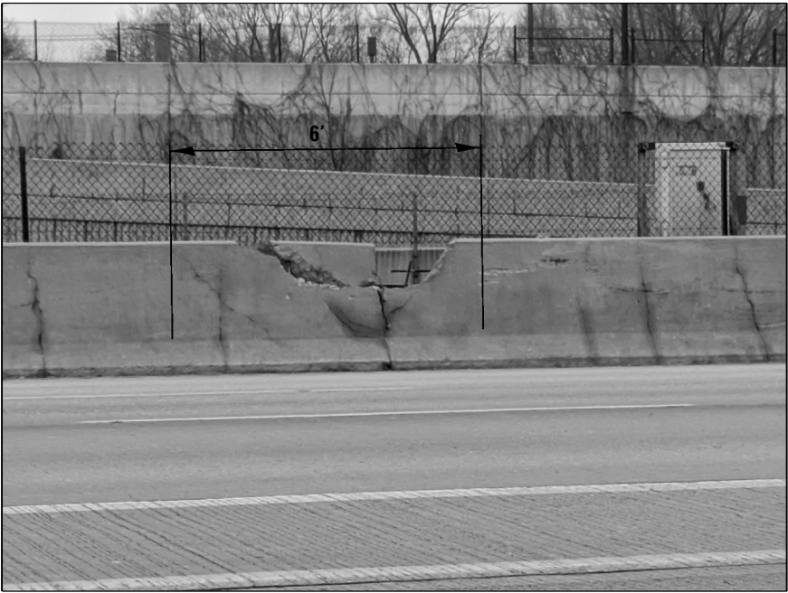
LOCATION 8. FULL DEPTH BARRIER WALL REPAIR REPLACE APPROXIMATELY 6 FT OF PARAPET LOCATED AT I-94 (DAN RYAN) SB LEFT SIDE AT 68th STREET
