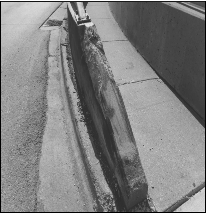
PARTIAL DEPTH PARAPET REPAIR LOCATED AT IL 171 SB NORTH APPROACH VERY NORTH END
