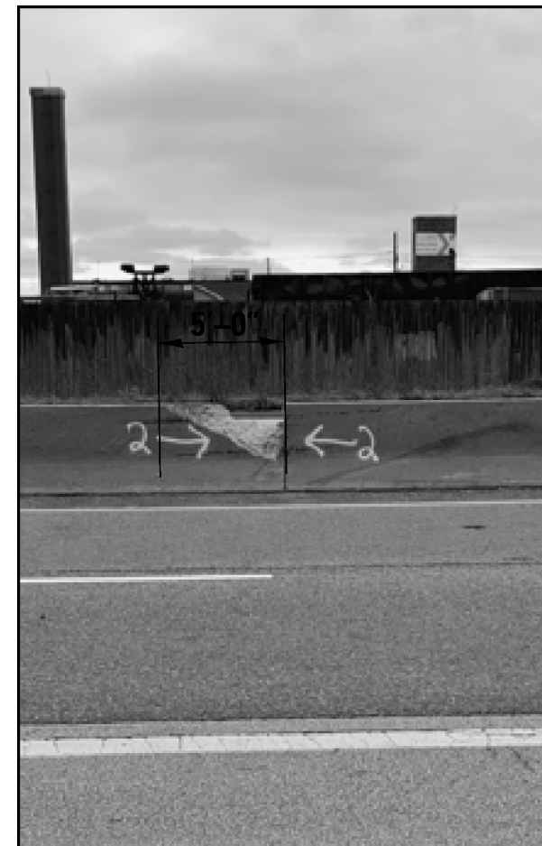
LOCATION 18. FULL DEPTH MEDIAN BARRIER WALL REPAIR REPLACE APPROXIMATELY 5 FT OF PARAPET LOCATED AT 120 FT WEST OF POPLAR CREEK IN ELGIN
