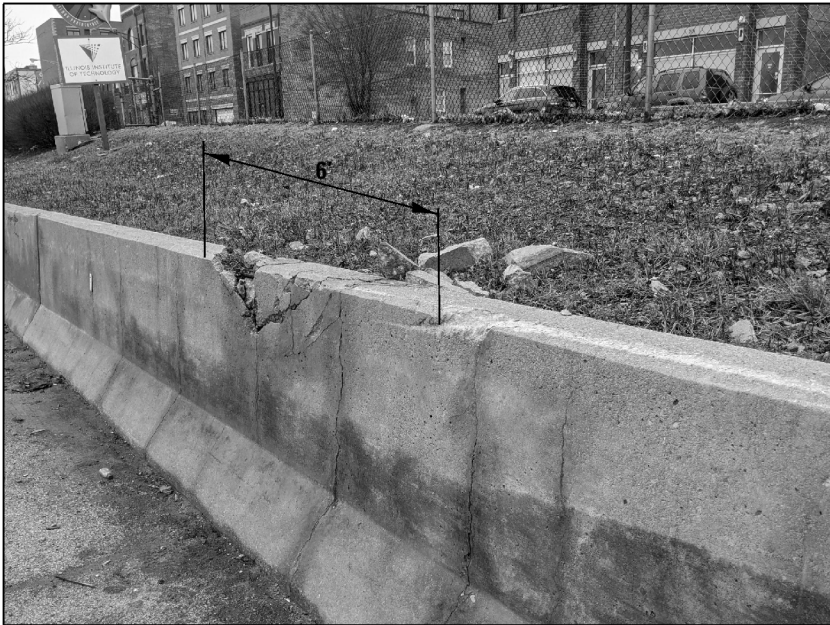
LOCATION 10. HALF DEPTH BARRIER WALL REPAIR REPLACE APPROXIMATELY 16 FT (2 SECTIONS) OF PARAPET LOCATED AT I-94 (DAN RYAN) SB LOCALS RIGHT SIDE JUST PAST 31st ST EXIT
