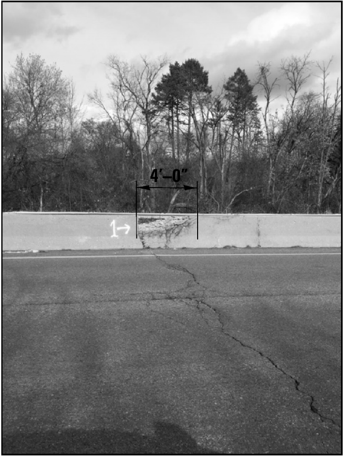
LOCATION 17. FULL DEPTH MEDIAN BARRIER WALL REPAIR REPLACE APPROXIMATELY 4 FT OF PARAPET LOCATED AT 120 FT WEST OF GRACE ST IN ELGIN
