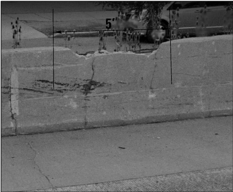
LOCATION 9. HALFL DEPTH BARRIER WALL REPAIR REPLACE APPROXIMATELY 6 FT OF PARAPET LOCATED AT I-94 (DAN RYAN) SB RIGHT SIDE LOCALS AT 29th STREET
