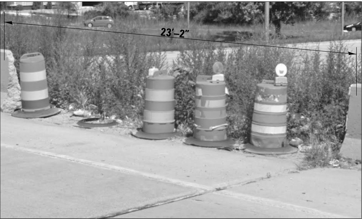
LOCATION 12A. FULL DEPTH BARRIER WALL REPAIR REPLACE APPROXIMATELY 23'-2" OF PARAPET LOCATED AT I-94 (BISHOP FORD FWY) NB AT DOLTON AVE RIGHT SIDE
