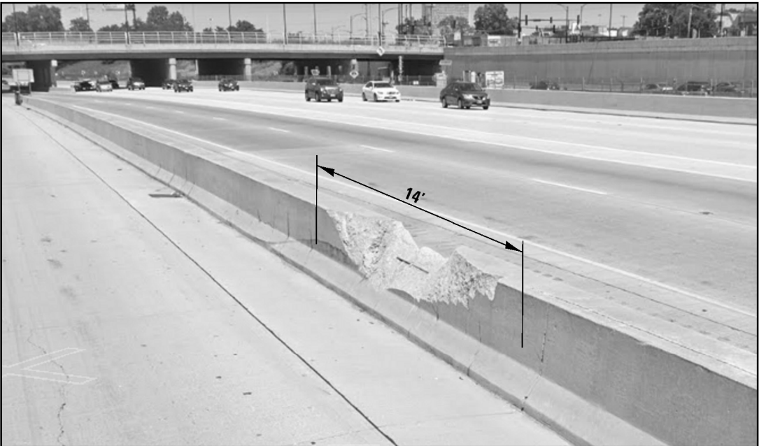
LOCATION 11. PARTIAL DEPTH BARRIER WALL REPAIR REPLACE APPROXIMATELY 14' OF PARAPET LOCATED AT I-94 (DAN RYAN) SB MEDIAN AT 68th STREET BETWEEN EXPRESSWAY AND RAMP
