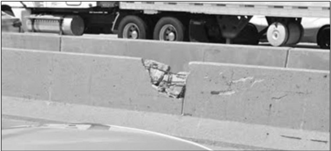
LOCATION 4A PARTIAL DEPTH PARAPET REPAIR REPLACE APPROXIMATELY 4 FT OF PARAPET LOCATED WEST SIDE, NORTH OF TRUSS OVER APPROACH SPANS
