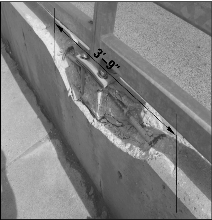
PARTIAL DEPTH PARAPET REPAIR LOCATED AT IL 171 SB NORTH APPROACH 26 FT SOUTH OF NORTH END
