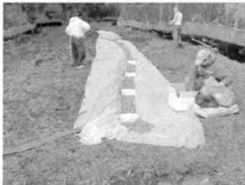
5) Apply Silt Stop (downstream end)
