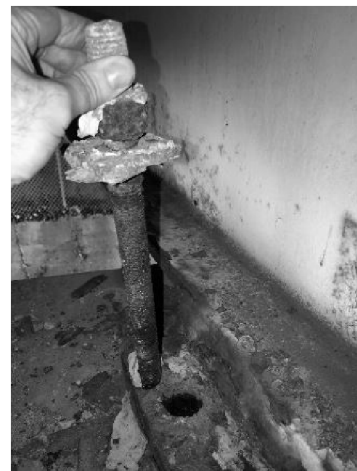
PHOTO 1: REPAIR ANCHOR BOLT
