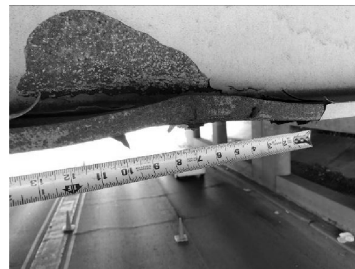
PHOTO 2: BEAM FLANGE REPAIR
