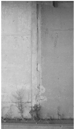
CRACKS ON PIER 2 (SF) (Looking North)
