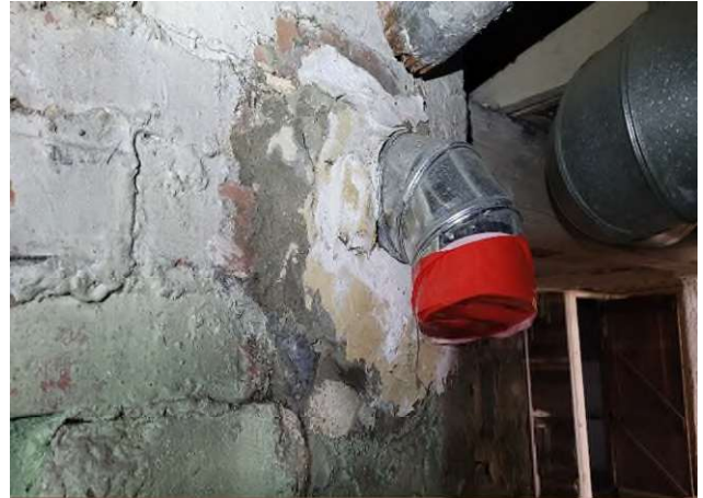
HA-22: White Chimney Flue Mortar (Patch) HA-23: Dark Gray Chimney Flue Mortar
