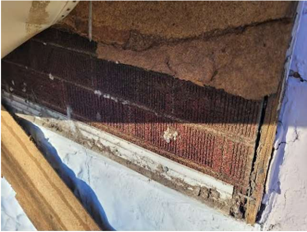
HA-29: Red/Black Asphalt Siding with Fiber Board Backing
