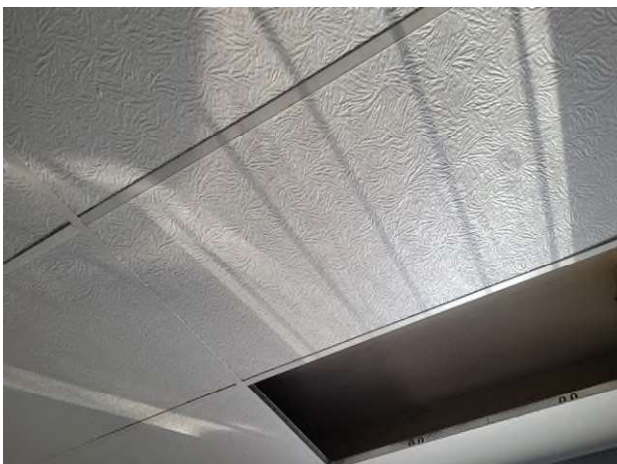
HA-4: White 2' x 4' Acoustical Ceiling Tiles (Smooth Wavy Texture)
