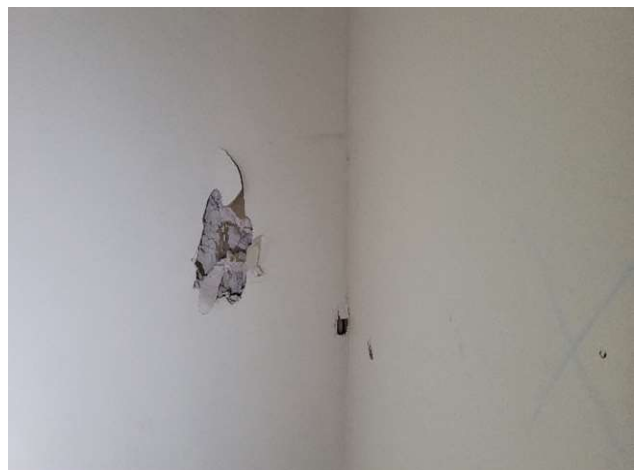
HA-18: White Gypsum Board HA-19: White Drywall Tape associated with HA-18 HA-20: White Joint Compound associated with HA-18
