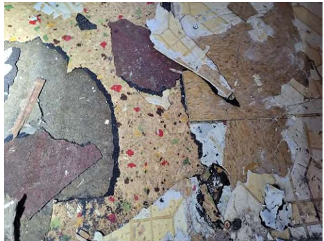
HA-15: Brown Linoleum with Red and Black Specks and Brown Paper Backing
