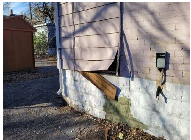
HA-28: Brown Wood Fiber Board behind Aluminum Siding
