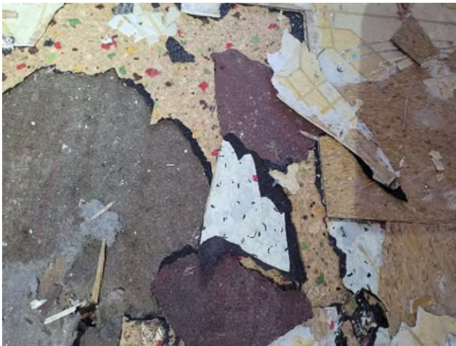
HA-14: White Linoleum with Black, Gray and Red Specks and Black Paper Backing
