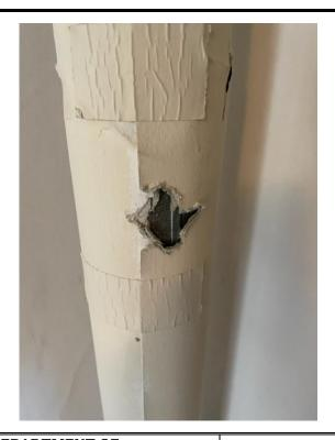
**Material Description:** Pipe Insulation - Tested **Positive for Asbestos**
