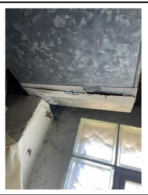
Material Description: Duct Wrap - Tested Positive for Asbestos
