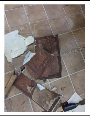
Material Description: Suspect ACM 12"x12" Wood Pattern Floor Tile and Mastic
