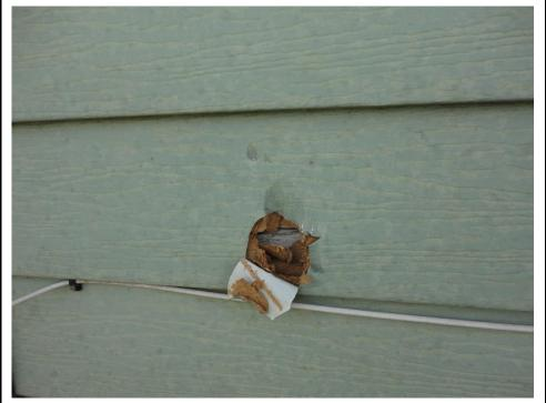
**Material Description:** Suspect ACM Wall Siding, Grey, Under AL Siding
