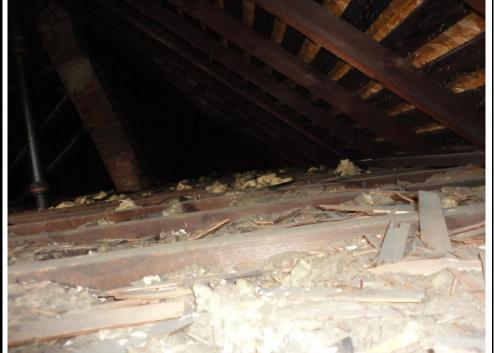
**Material Description:** Suspect ACM Attic Floor Insulation
