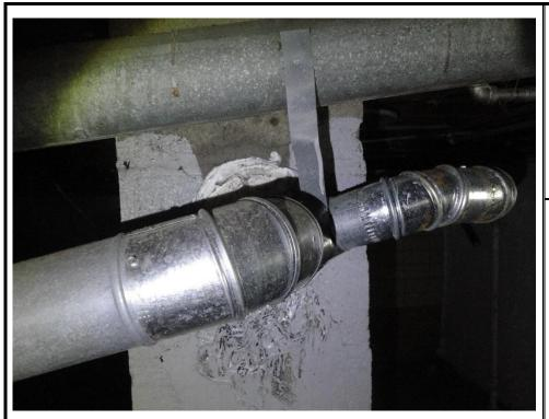
**Material Description:** Suspect ACM Concrete Wall Seal
