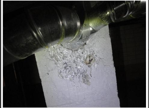
**Material Description:** Suspect ACM HVAC Insulation/Seal, Grey
