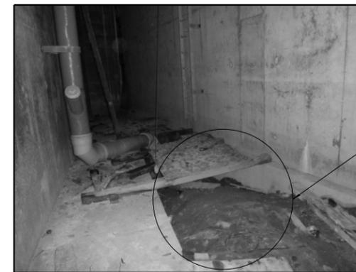
Backfill soil up to the level of existing ladder. Cost to be included with Debris Removal.
