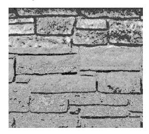
The retaining wall shall be constructed with a coursed stone rusticated surface with a 1" relief. The aesthetic surface treatment shall be accomplished by the use of form liners as specified. The walls shall not contain patched or unpatched tie holes. The concrete pours shall be coordinated to prevent visible differences between individual pours or batches.
